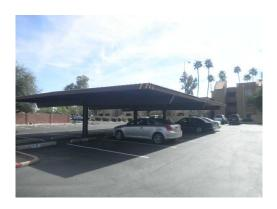
Approximate 223,350 sf of driveways and parking areas. Resurfaced in 2006 for a total of \$234,360. If asphalt is maintained properly and assessed frequently this asset's useful life may be able to be extended.
