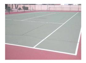
Poor condition. Badly cracked. Replace one court. Cost assumes using post-tensioned concrete which should last indefinitely.
