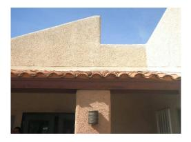
Approximately 2030 sf replacement of underlayment with 2 layers of 30# ASTM felt by USA Roofing.
